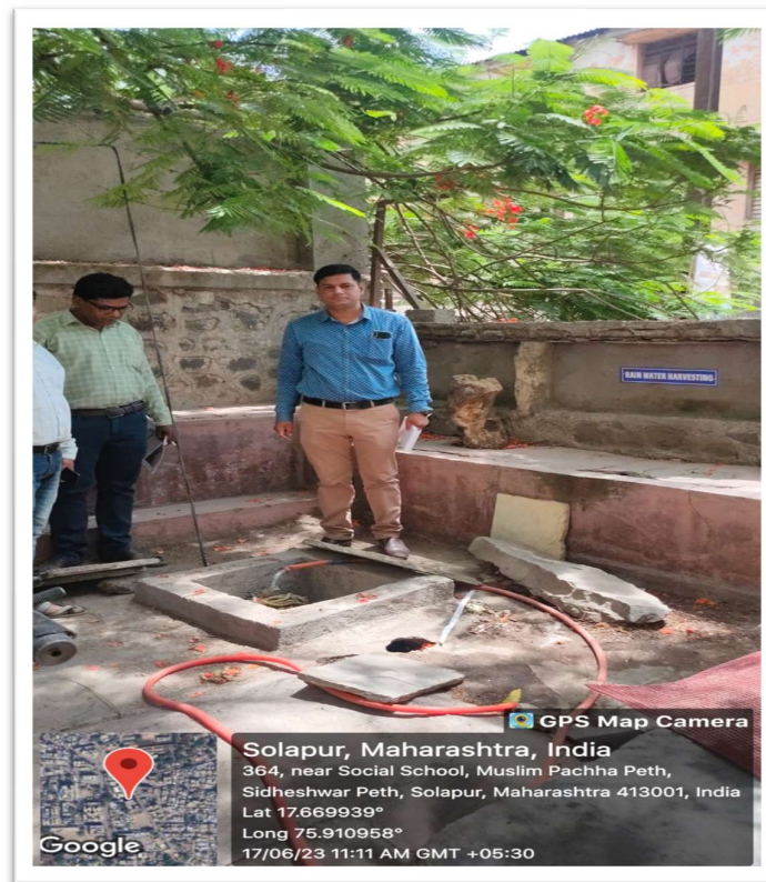
Fig.32: Rain water Harvesting – Water Recharging through Borewell
